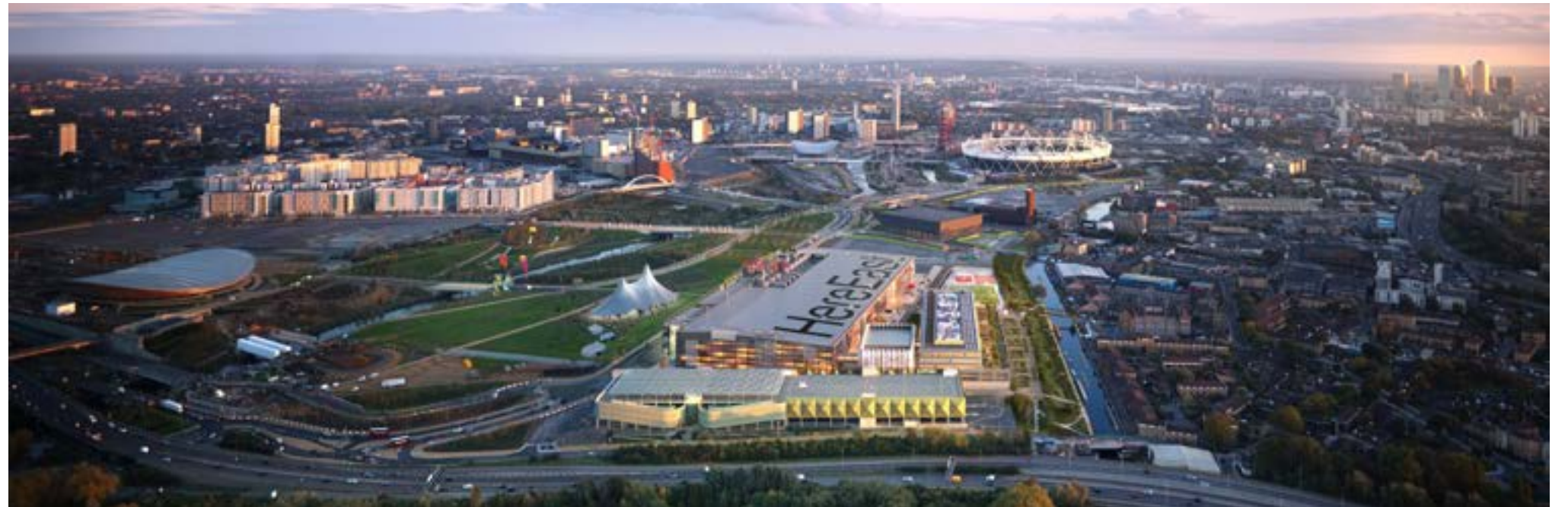
Here East Olympic Park - London
