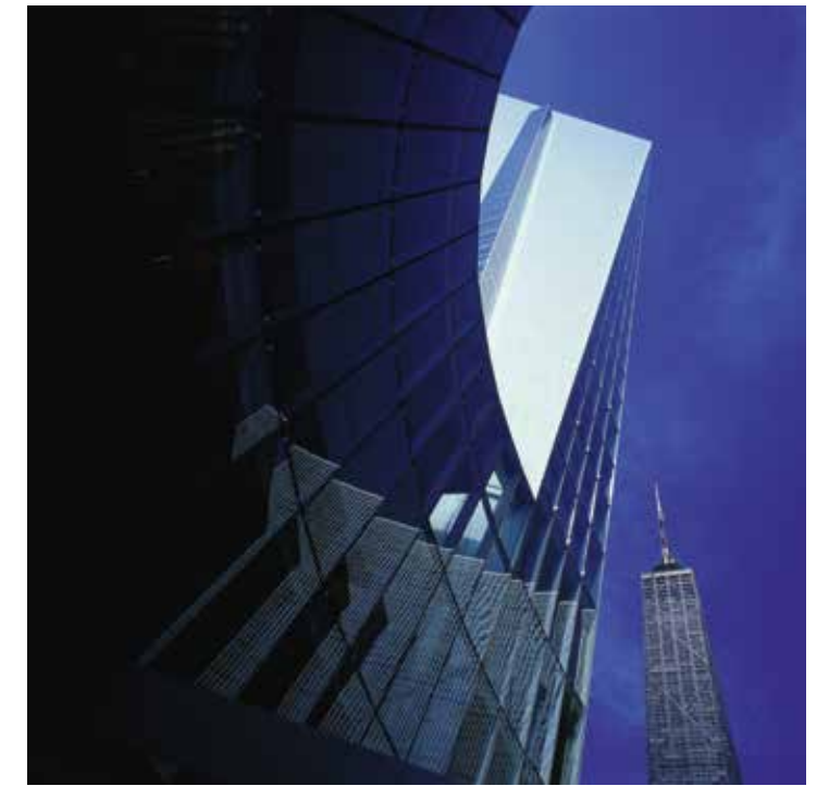
Exterior, Sofitel Chicago Water Tower, Chicago, USA
