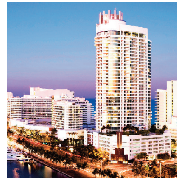
FONTAINEBLEAU TRESOR TOWER, MIAMI BEACH, FLORIDA
